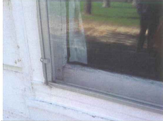
Photo #2: Exterior House, Window Glazing
