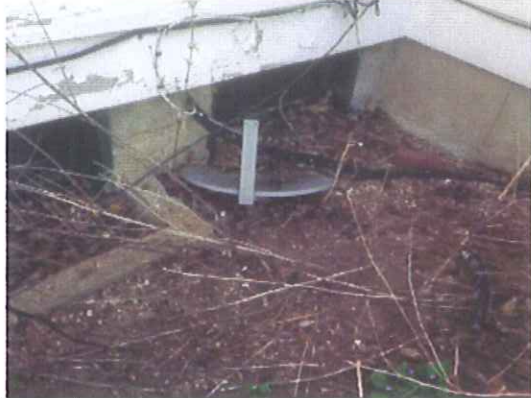
Photo #1: Exterior House, Window Glazing
