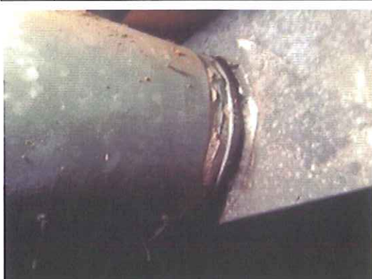
Photo #5: House Interior, Duct Tape (Mainly Basement)
