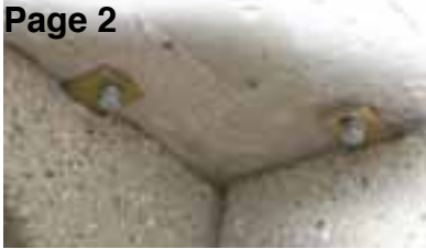
Step 12 Snug bolts. Do Not Over Tighten
