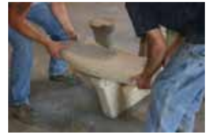
Step 16 Install seats. Carefully lower seats on top of angles
