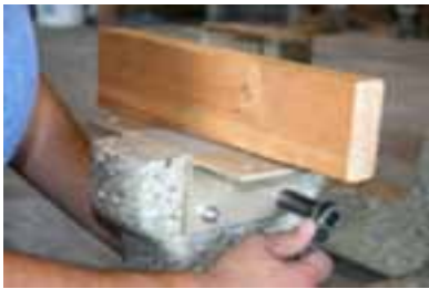
Step 15 Make sure angles are flush (or slightly above) the top of concrete legs. Use a straight edge or 2 x 4 to help line up. Make sure angles on four legs are flush and secure. Do Not Over Tighten
