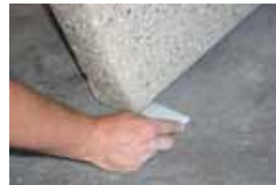
Step 19 Shim legs. If table teeters shim bottom of legs until steady.
