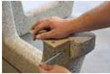
Step 13 Assemble seat angles. Use 3/8"-16 X 5" Hex head cap screw.
