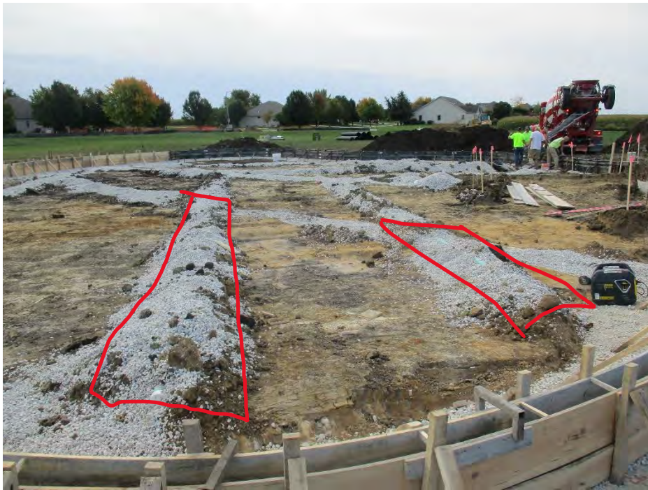
Two sections of drain pipe to be removed by the GC.
